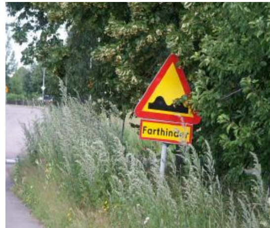
Figure 2.21 Bad Sign Positions (partially occluded signs)
