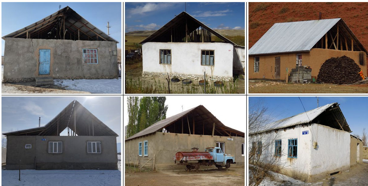
Fig. 3 Typical rural Kyrgyz houses with natural walls and open gable roof
